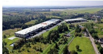
7R CITY FLEX KRAKÓW AIRPORT
