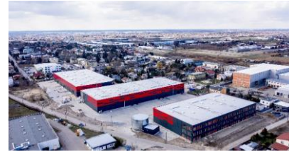
7R CITY FLEX WARSAW AIRPORT I
